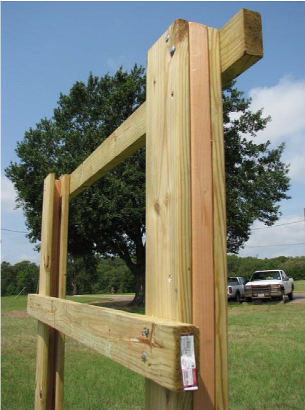
Upper Left-Gate Frame (note cross brace 4' above the ground faces inside of trap)
