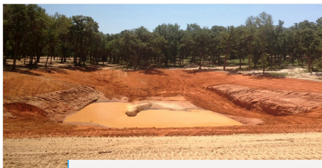
Figure 1. Newly constructed pond illustrating construction in clay soils. Photo displays how clay particles easily become suspended as the pond begins to fill, creating turbid or muddy water.
